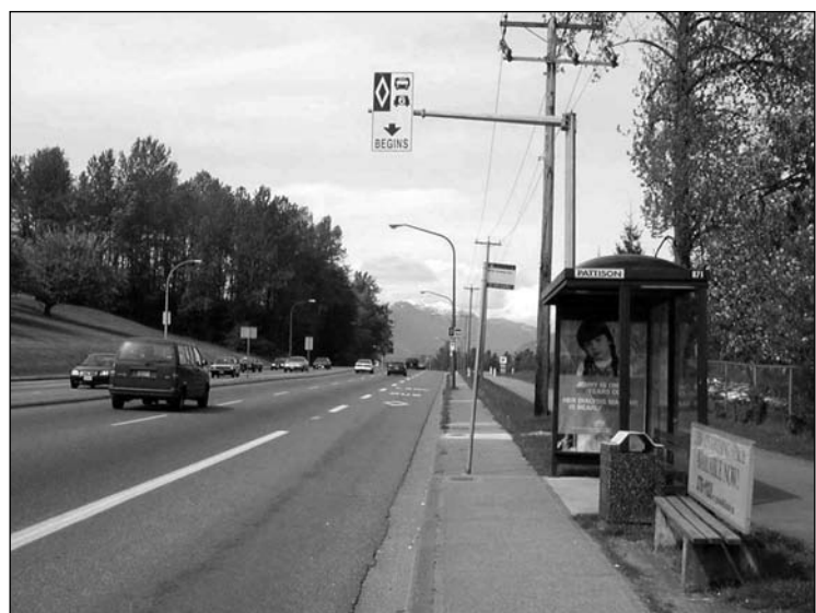
Figure 3–10: Typical HOV Lane
