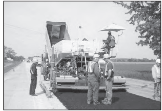
b) Paving of first 70 mm lift of cold recycled asphalt
