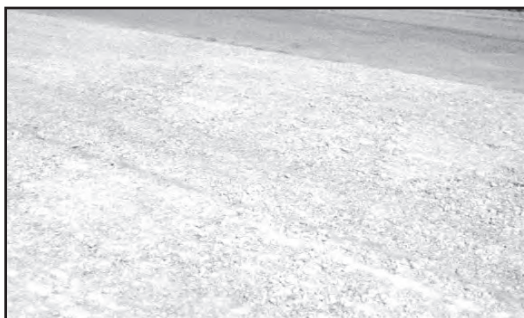
b) Surface appearance of the rubblized PCC before compaction.
