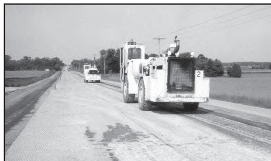
a) Pulverization of PCC using three IRB resonant breakers working in echelon.
