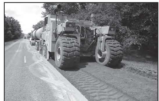
Photo 3-9: Full depth reclamation with cement stabilization
