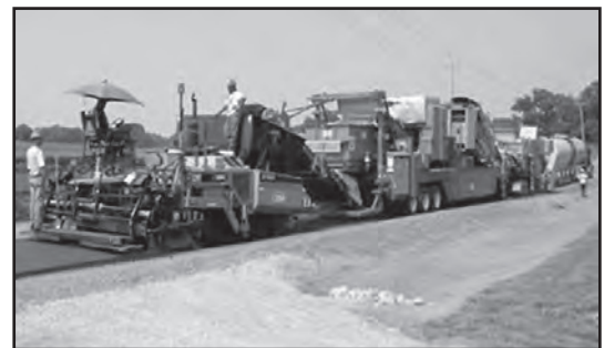
Photo 3-7: Paver-Laid surface recycling foamed asphalt train (Adapted from SOTER Technology)
