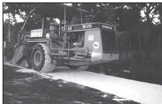
Photo 3-8: Full depth reclamation with lime stabilization
