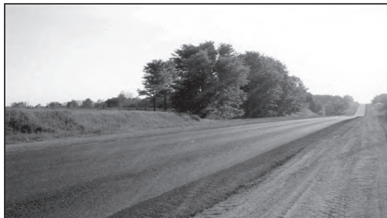
Photo A-3: View of Completed Oxford County Road 2 Project
