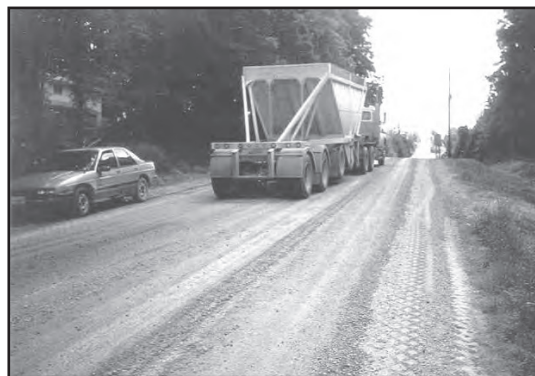
a) Placing additional granular material on top of pre-pulverized old pavement.
