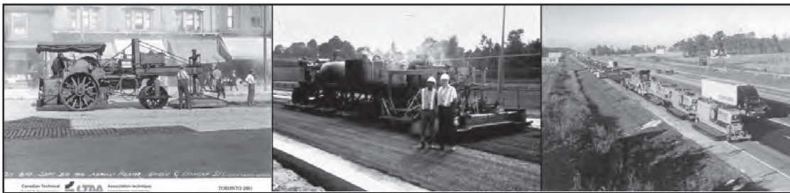
Photo A-9: Hot in-place recycling and equipment used, past and present
