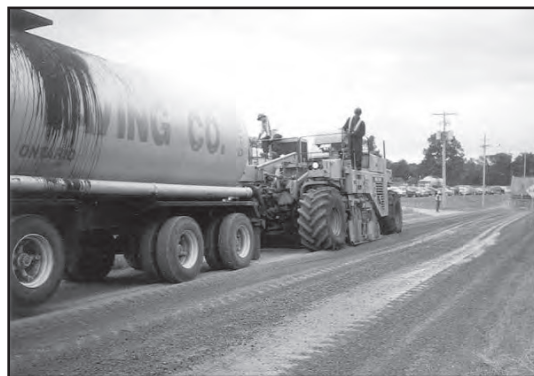
b) 150 mm of foamed asphalt stabilization asphalt cement at 150°C plus 2% water.
