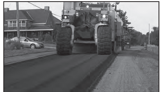
Photo 3-6: Conventional full-depth foamed asphalt stabilization unit
