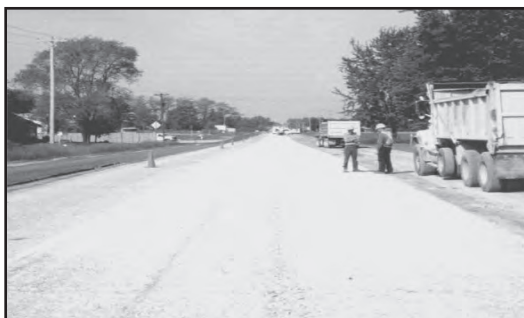
d) Appearance of rubblized and compacted Oxford County Road 2.
