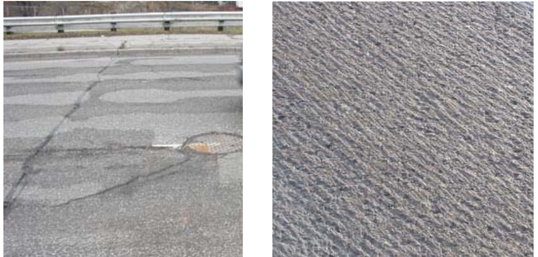
Figure 3–19: Micro-milling application to reduce rutting and roughness. The milled surface has darker colour (a). The milled surface on the right (b) has grooves with the peak to peak distance of about 15 mm.
