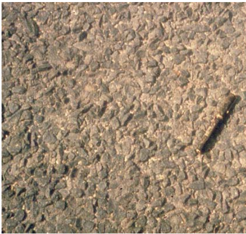
Figure 3–14: Surface of a newly constructed seal coat using 13.2 mm chips and CRS-2P emulsion
