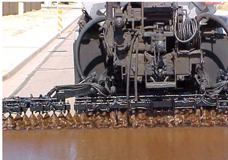
Figure 3-13: Asphalt distributor applying emulsion; view from the back. The emulsion has a typical brown colour which changes into black colour as the emulsion cures. Nozzles on the spray bar provide good coverage of the surface.
