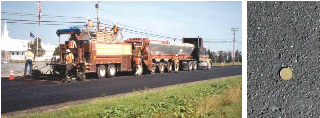
(a) (b) Figure 3–7: Truck-mounted self-propelled continuous feed micro-surfacing machine (a); surface texture (b).
