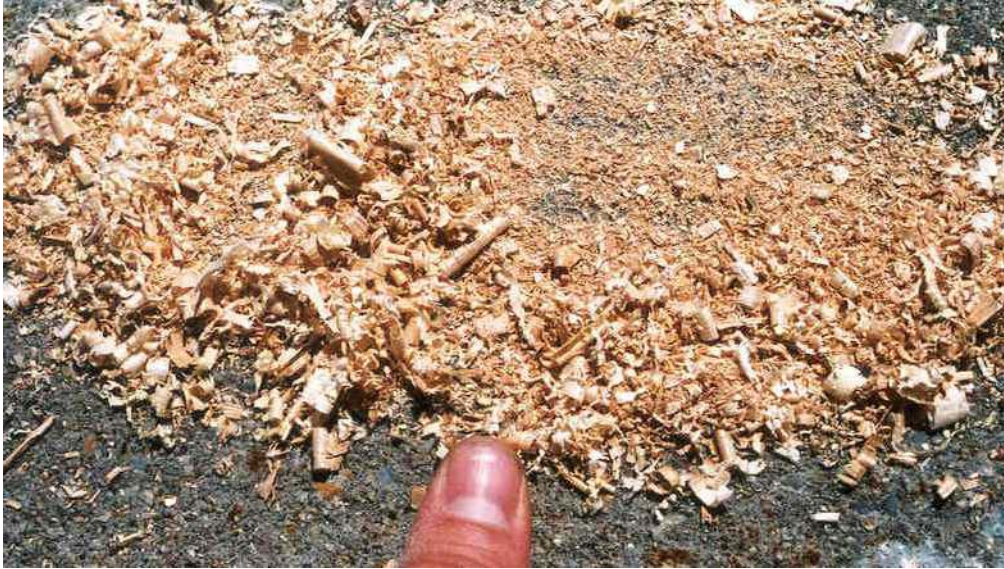
Photograph 3–4: Fine wood shavings to protect hot sealant from tires
