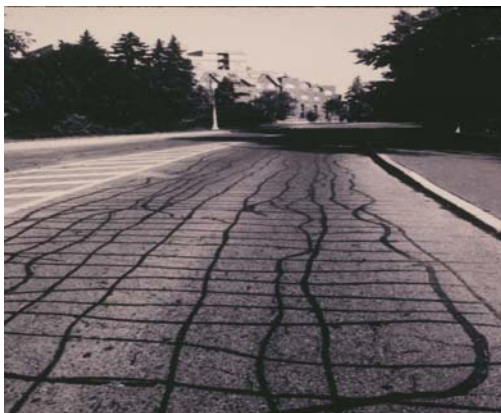
Figure 2–2: Pavement sections unsuitable for crack sealing
