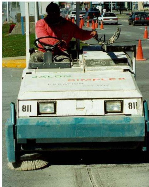
Photograph 3–2: A mechanical sweeper cleans away routing dust
