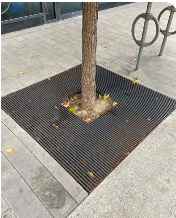
FIGURE 6: METAL TREE GRATE ON A BOULEVARD
