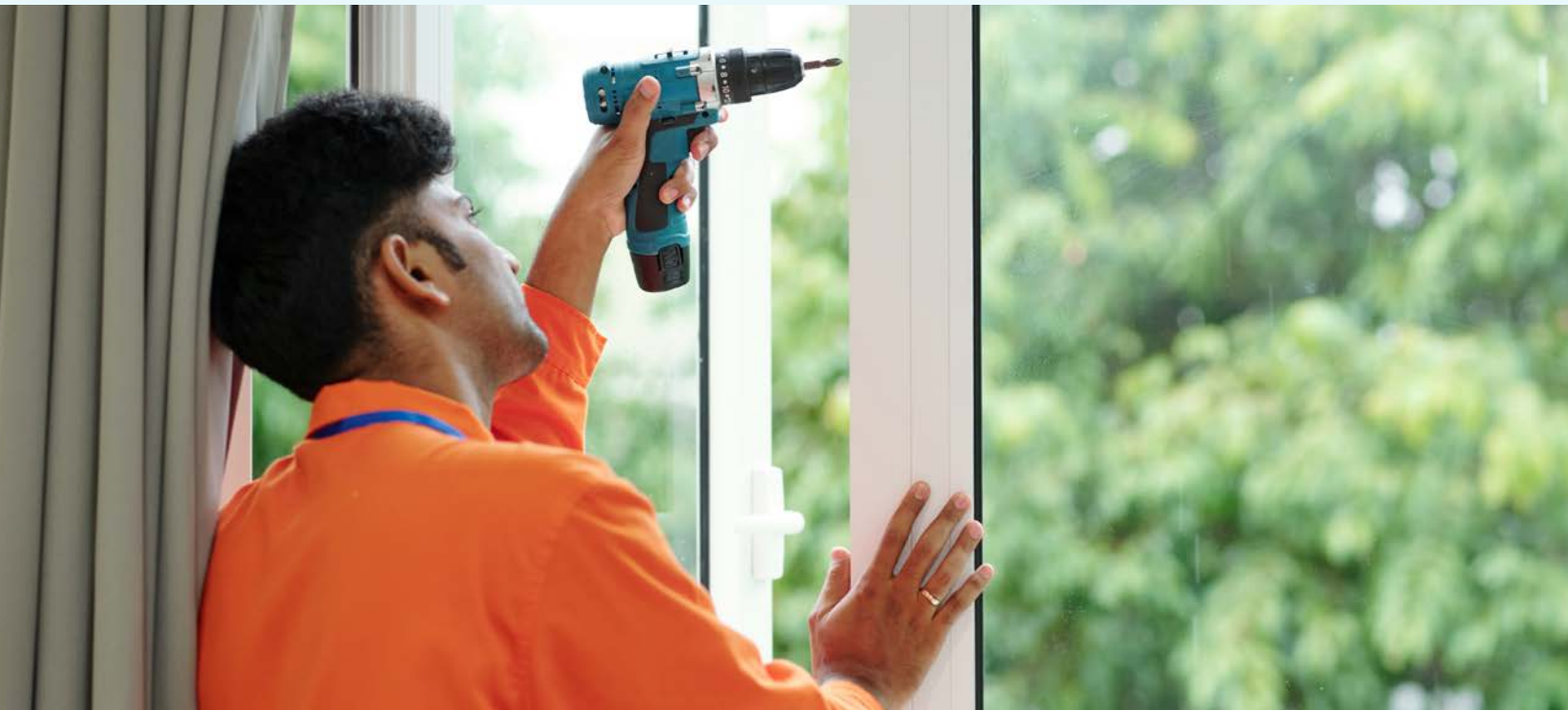
Construction workers installing windows
