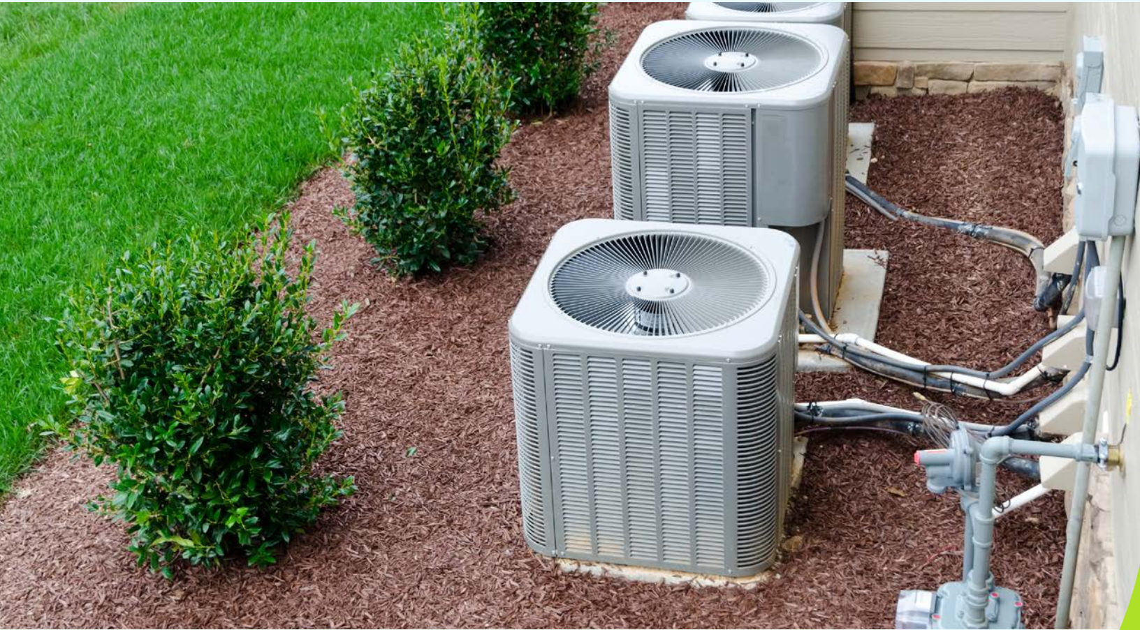
AC units connected to the residential house
