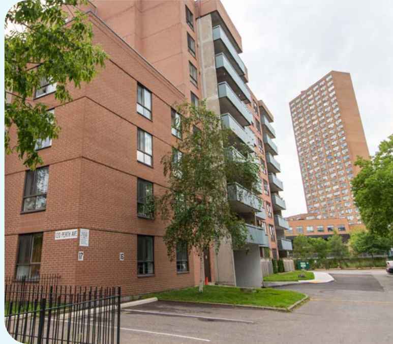
Perth Avenue Housing Co-operative Photo courtesy of The Atmospheric Fund (TAF)
